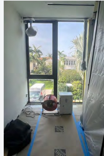
Industrial dehumidifiers and tarp deployed in child's room
