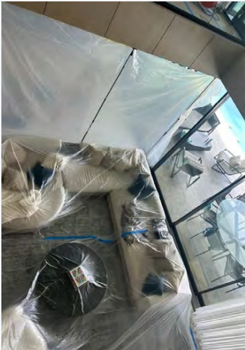
Tarp covering entire living room during remediation
