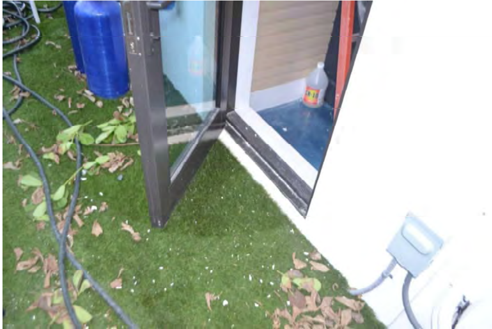
Figure 59) View showing exterior grade elevation near door threshold at the left elevation of the home.
