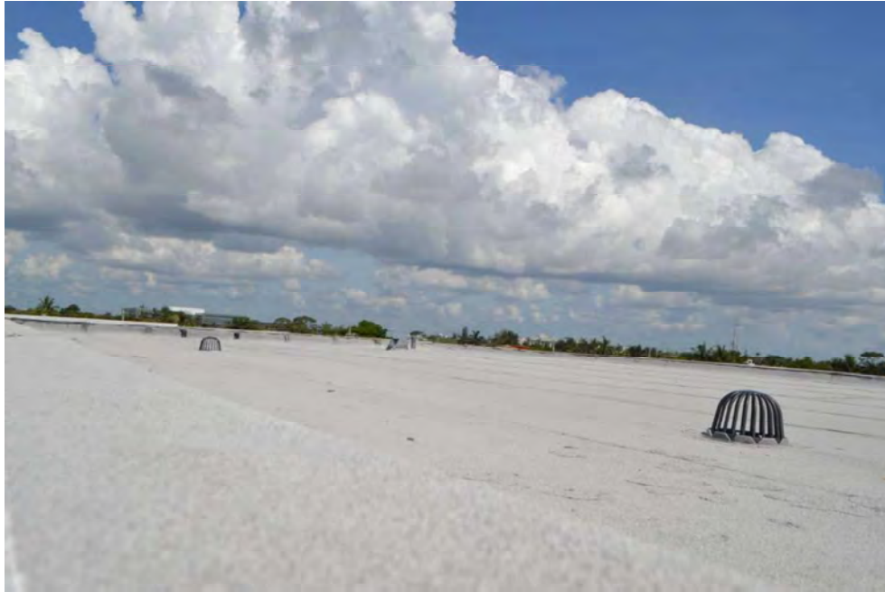
Figure 27) Overview of the upper roof covering.
