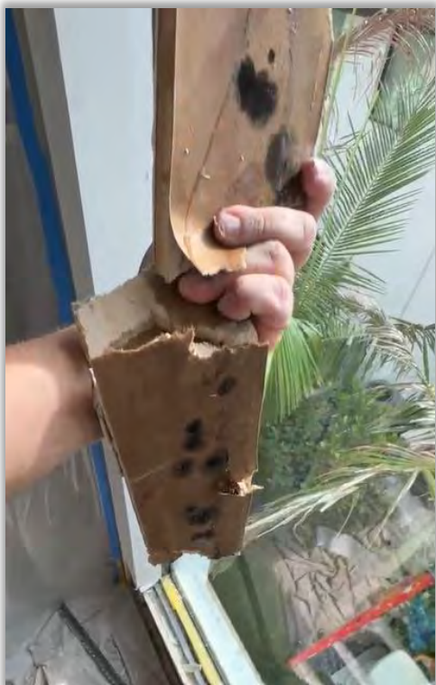
Figure 3: Black mold growing on drywall in daughter's room.
