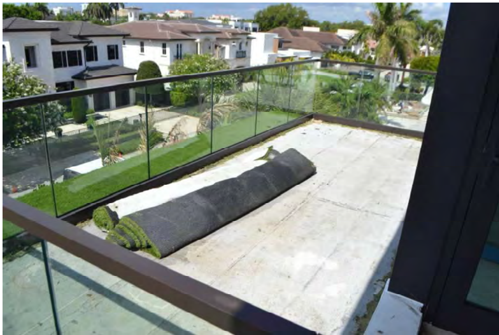
Figure 20) Overview of the front roof at the third floor.
