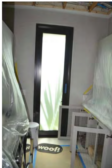
Figure 46) Overview of the laundry room.
