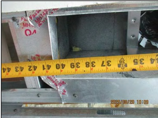
Length of diffuser measures 41-inches
