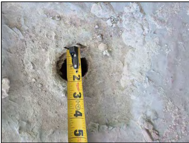
Drain outlet of 2-inches
