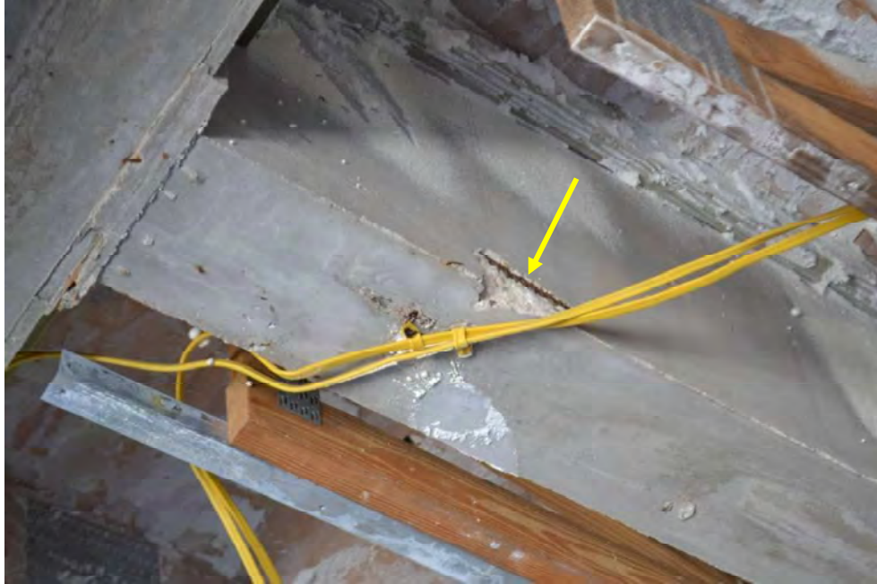
Figure 49) View of spalled concrete and inadequate rebar clearance at a beam above the garage.
