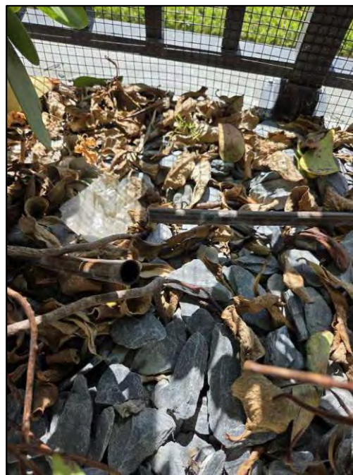
Disconnected irrigation drip lines at the perimeter planters
