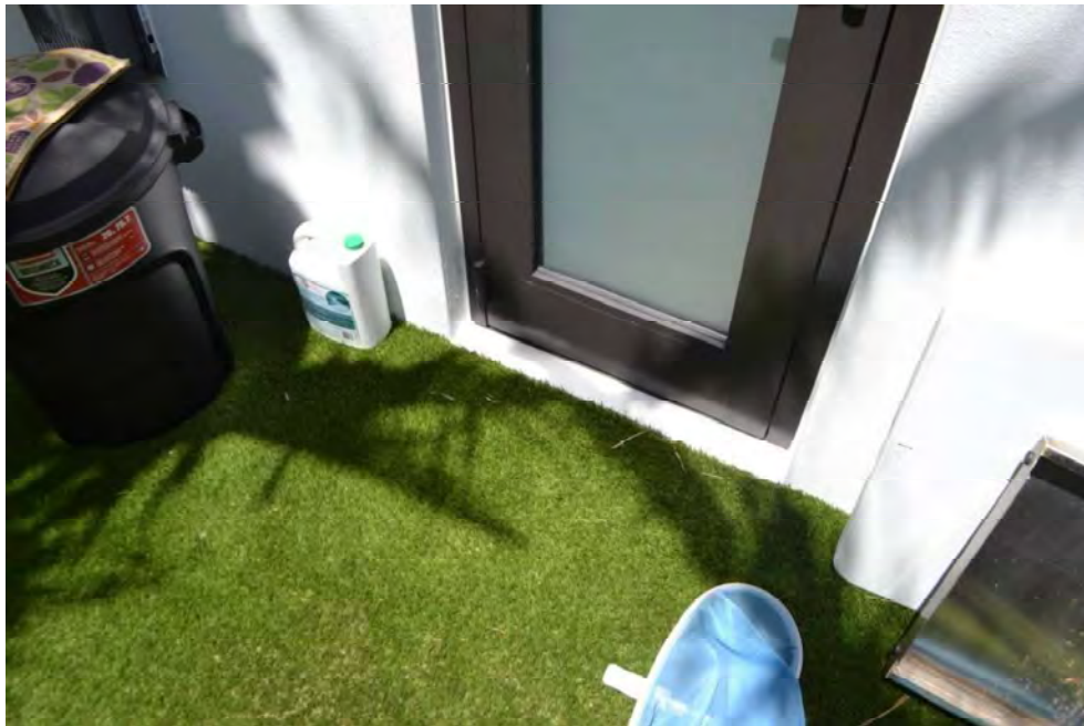
Figure 62) View showing exterior grade elevation near door threshold at the right elevation of the home.
