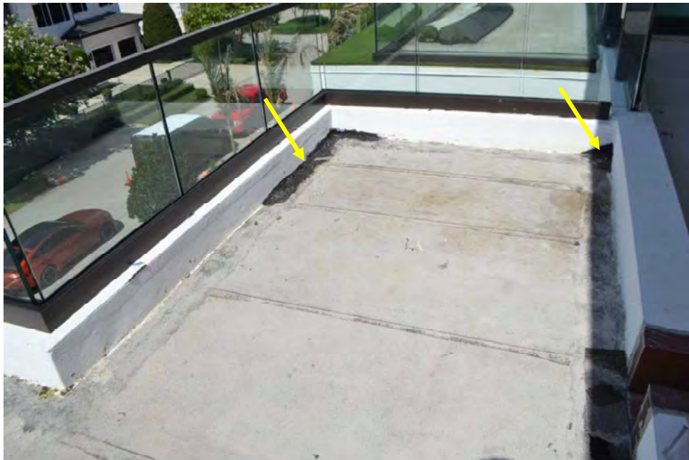
Figure 26) Exemplar view of recent roof repairs observed at the front third floor roof.
