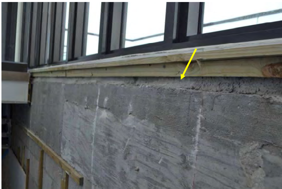
Figure 10) View of low-strength grout installed between the window buck and concrete beam at the stair to the third floor.
