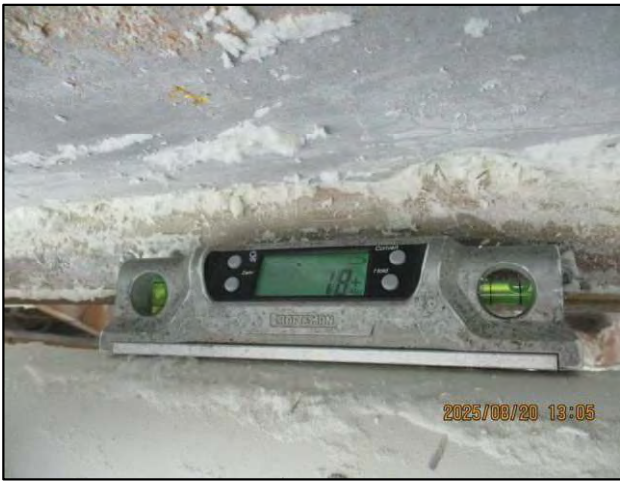
Reverse pitch observed on the storm drainage piping
