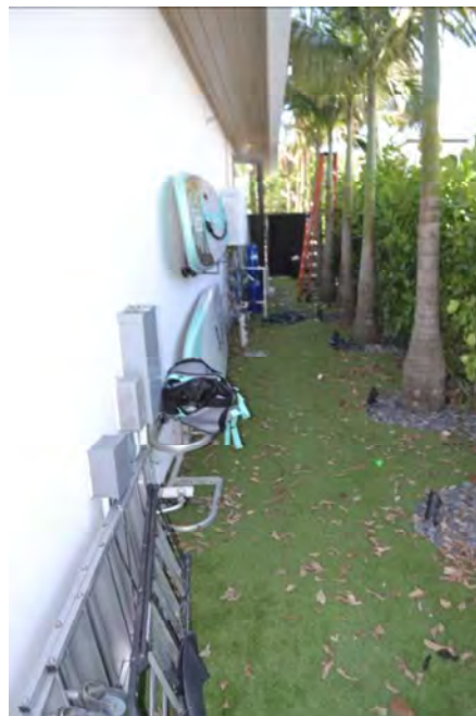
Figure 58) Partial view of the left elevation of the home.
