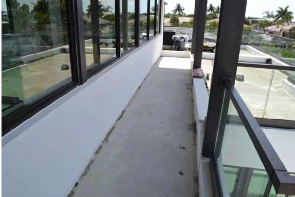
Figure 21) Overview of the front third floor balcony.
