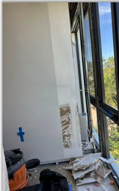
Figure 4: Damage to children's rooms by water intrusion through windows.
