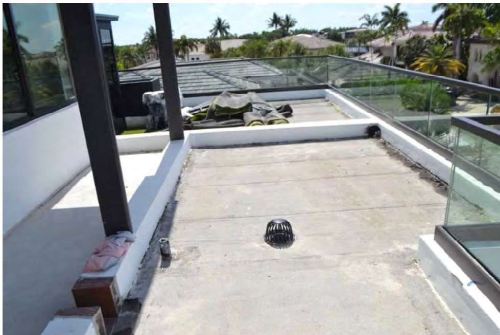
Figure 22) Overview of the front roofs at the third floor.
