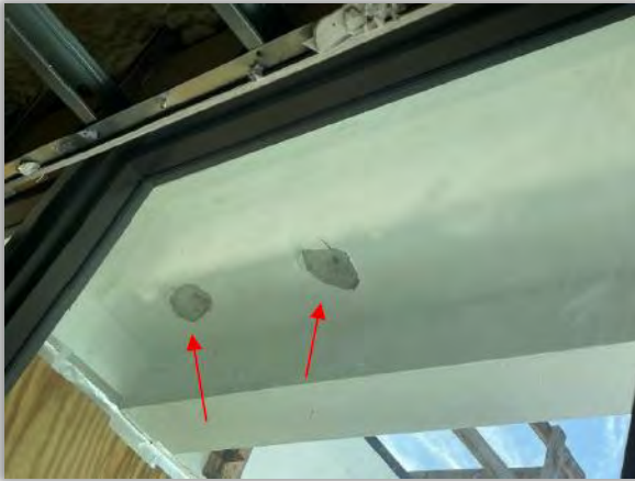
Figure 15: holes drilled through balcony slab to drain ponding water
