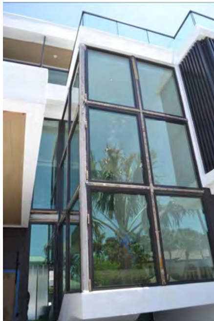
Figure 2) View of the exterior walls of the main stair.
