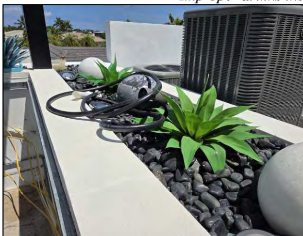
No provisions of overflow drainage in outdoor terrace planters
