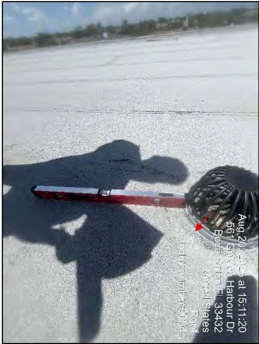
Photo 9004: Measurement of 0 % slope on roof at 4 th Floor.
