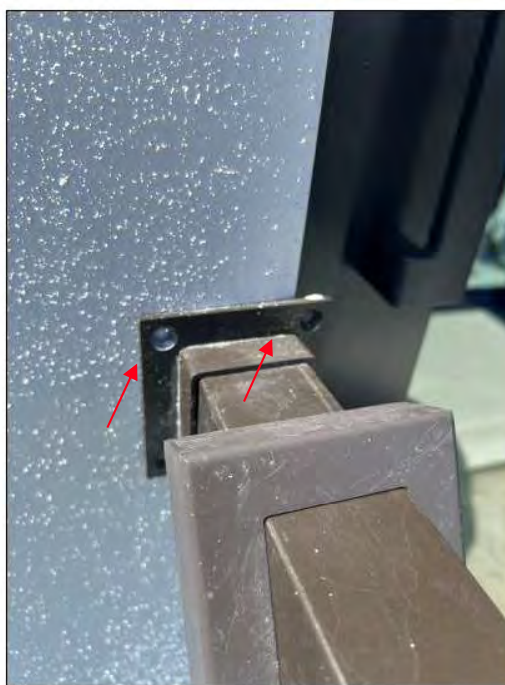
ECS Photo 24 – Missing fasteners at railing system. Also, railing end location is incorrect as it is not completely supported by the structural substrate.
