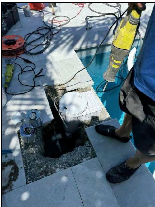
Excavation of the installed skimmer at the pool
