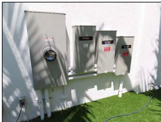
Automatic Transfer Switches
