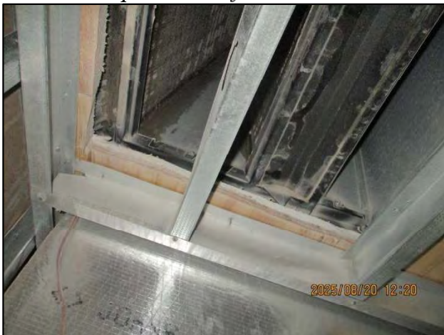
Typical construction of the return air plenum box support with drywall and metal wall studs.
