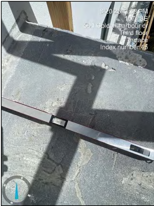
Photo 45: Third Floor Terrace – General view of the north terrace without any slope.
