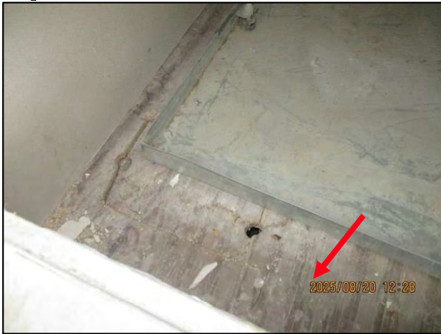
AHU #1 plywood sheet installed within return air plenum.
