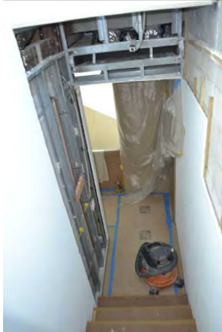
Figure 7) Overview of the stair to the third floor.
