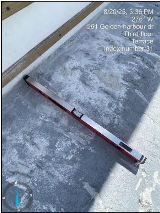
Photo 31: Third Floor Terrace – General view of the north terrace without any slope.
