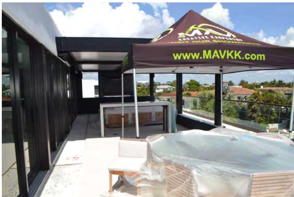
Figure 13) Overview of the third floor rear balcony.
