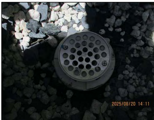
Improper drains installed in the planter
