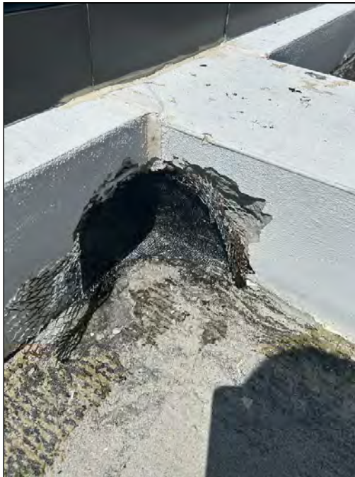
10 - Roofing level pending remediation and stucco application.
