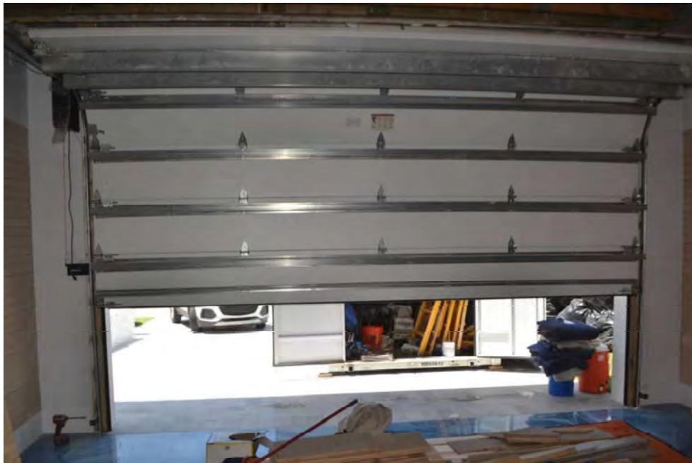
Figure 48) Overview of the garage.
