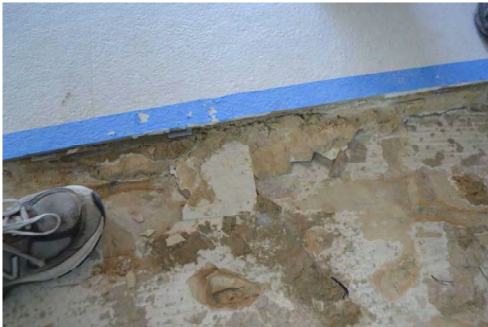
Figure 30) View showing pavers installed over a tile floor.
