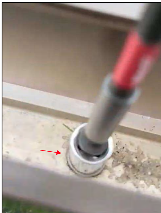
561-6.5.25- Video#1 Still 1 – Showing general view before removal of unsealed fastener from railing system base channel.
