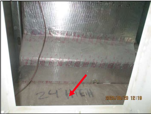
AHU #2 plywood sheet installed within return air plenum.
