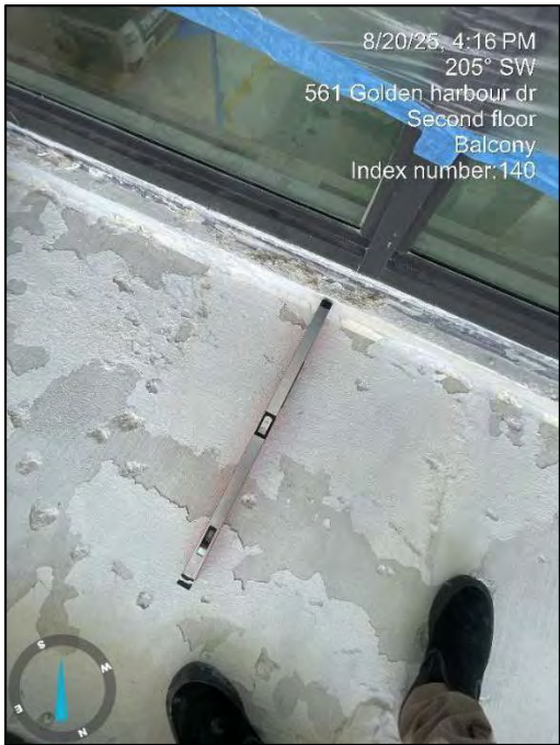
Photo 140: Second Floor Balcony – General view of the north balcony without any slope.
