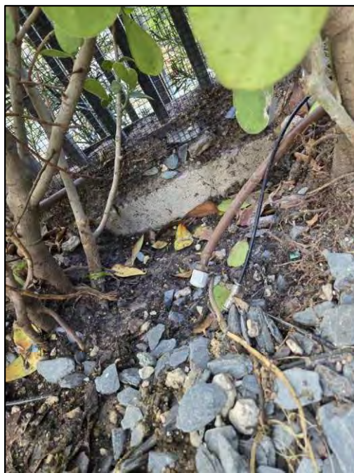
Disconnected irrigation drip lines at the perimeter planters
