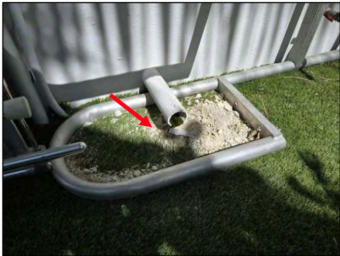
Typical conditions of rainwater drainage piping missing splash block and obstructed
