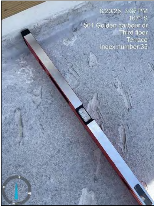
Photo 35: Third Floor Terrace – General view of the north terrace without any slope.
