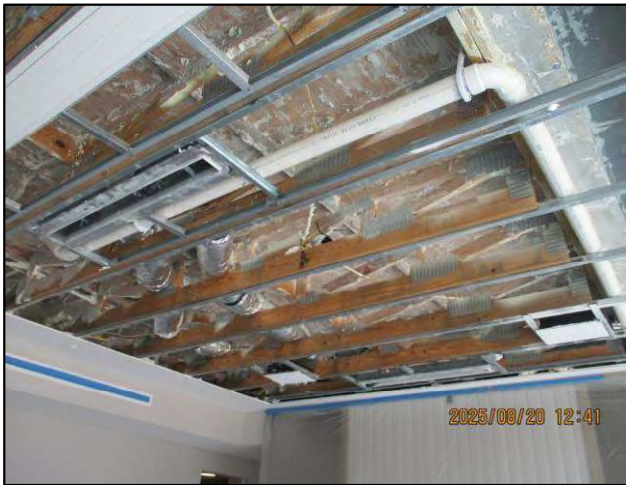
Reverse pitch observed on the storm drainage piping
